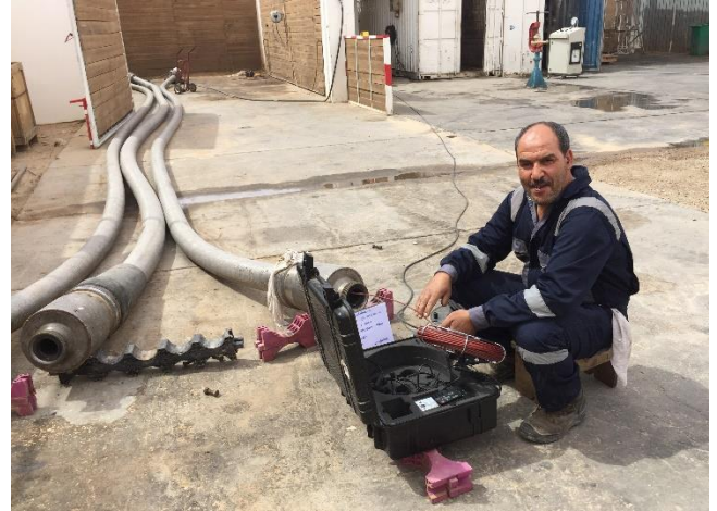
Camera inspection in HP hose.
